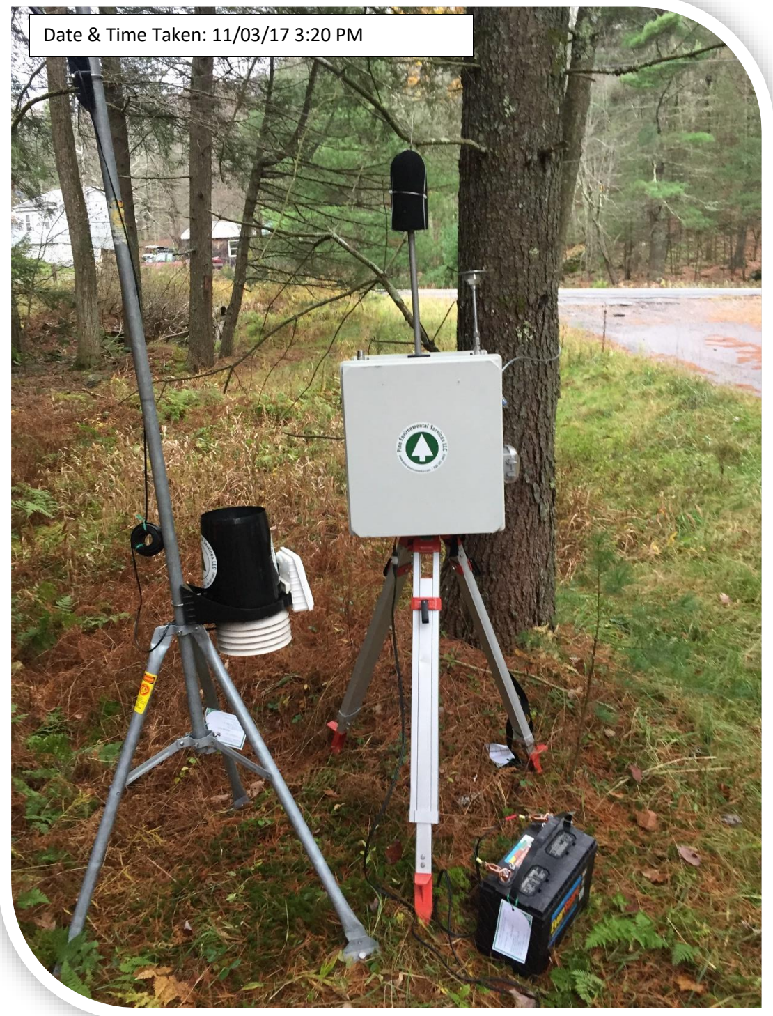
Figure 5: Telemetry Set Up and Weather Station in Location 6, Powered by a Marine Battery
