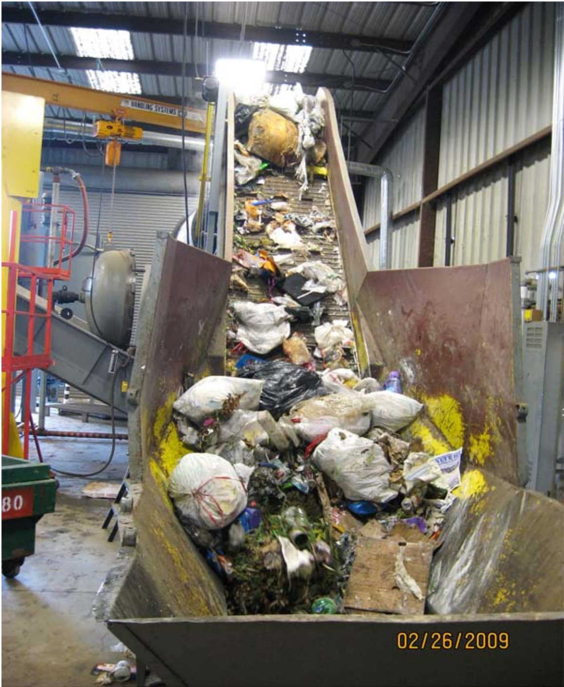
Figure 2 The autoclave being loaded with waste
